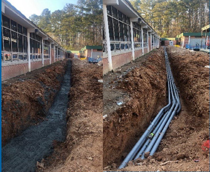
Concrete Encased Conduit to Transformer Pad
