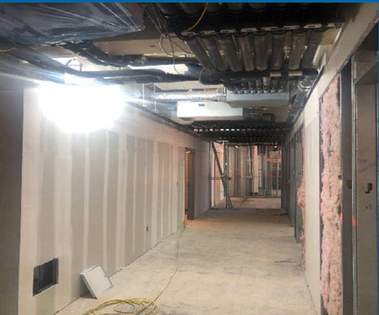
Admin Area MEP OH and Finished Drywall
